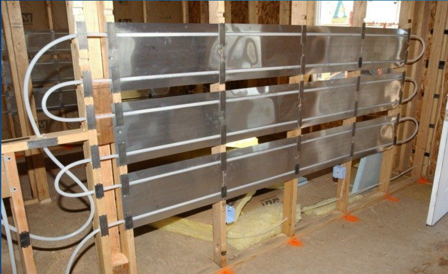
Figure 6: In-wall radiant heating in a home [27]
